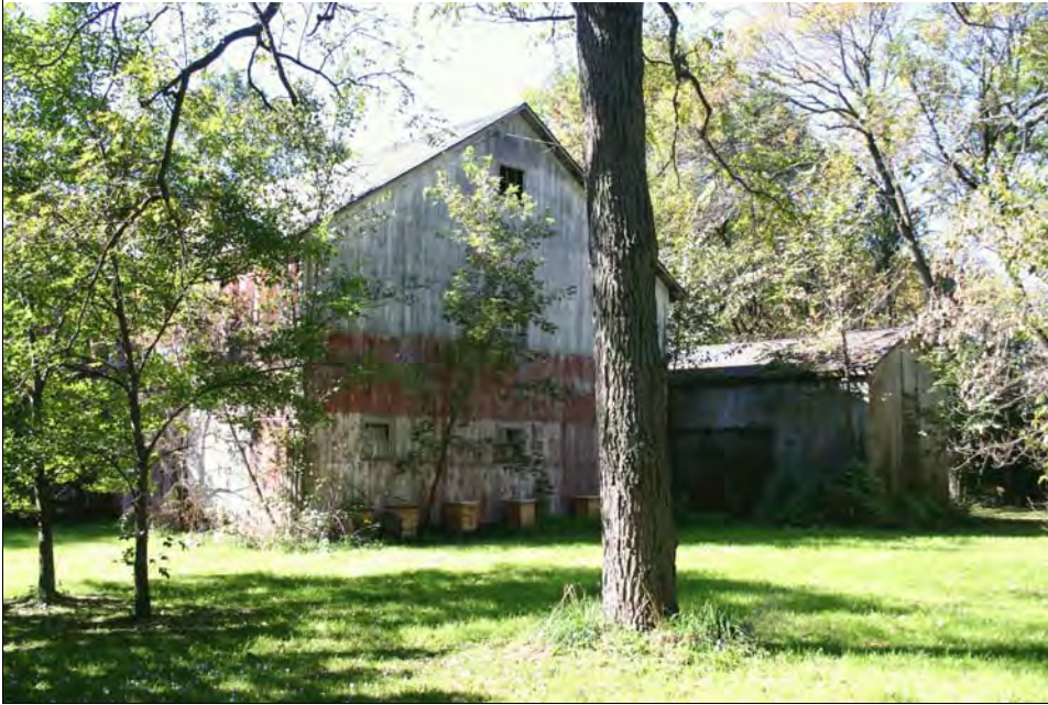
Figure 8: Barn and adjacent Outbuilding. View to south southwest.
