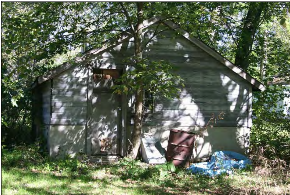
Figure 7: Storage Shed. View to north.
