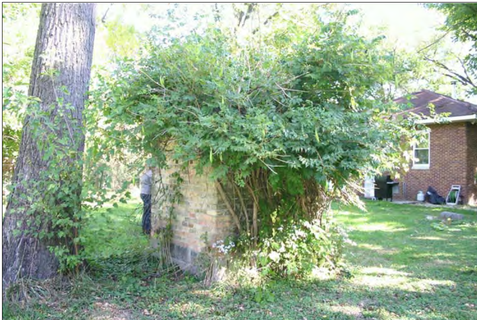
Figure 5: Outhouse. View to northeast.
