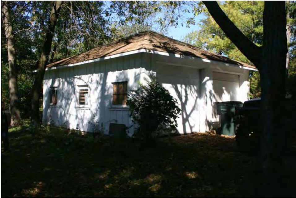
Figure 6: Garage. View to northwest.
